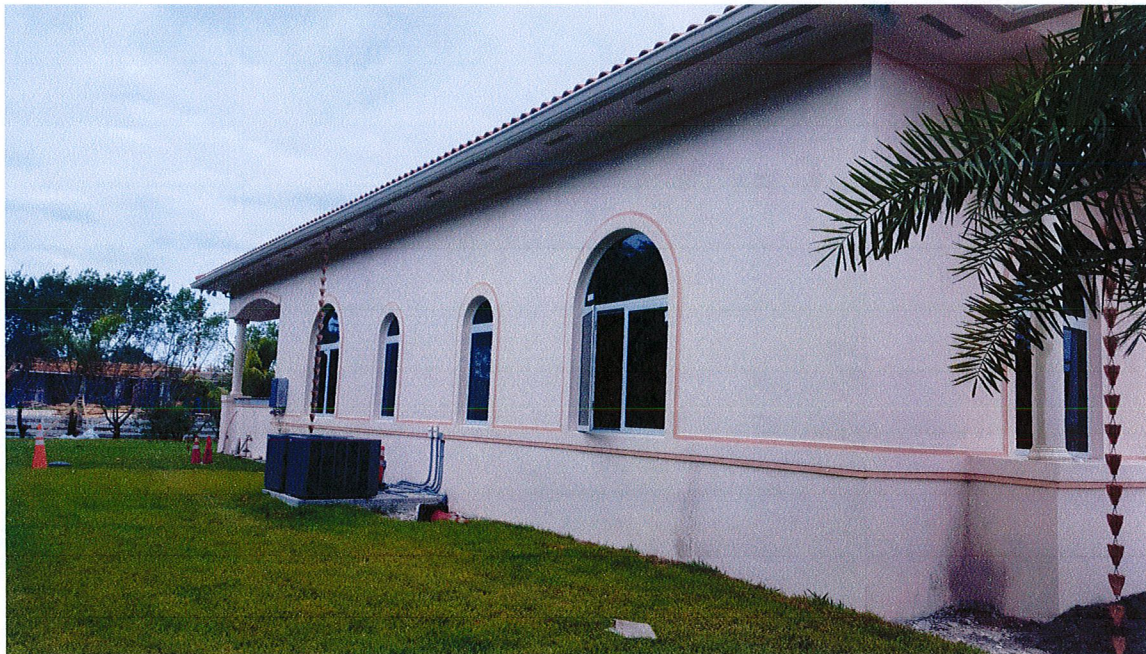
LEFT SIDE OF PROPERTY (SOUTH SIDE)
