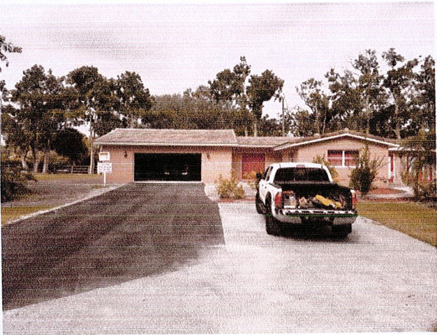
FRONT VIEW LOOKING NORTHERLY
