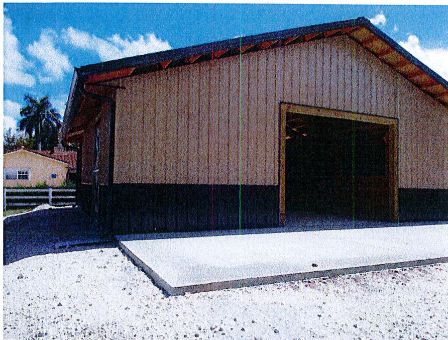
REAR OF STABLE 5/27/16
